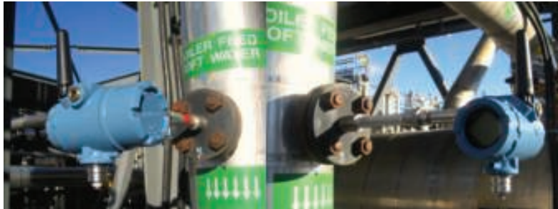
FIGURE 3. These modern wireless temperature transmitters have been successfully operating in Fort McMurray, in Alberta, Canada, for several years, without the need for enclosures
